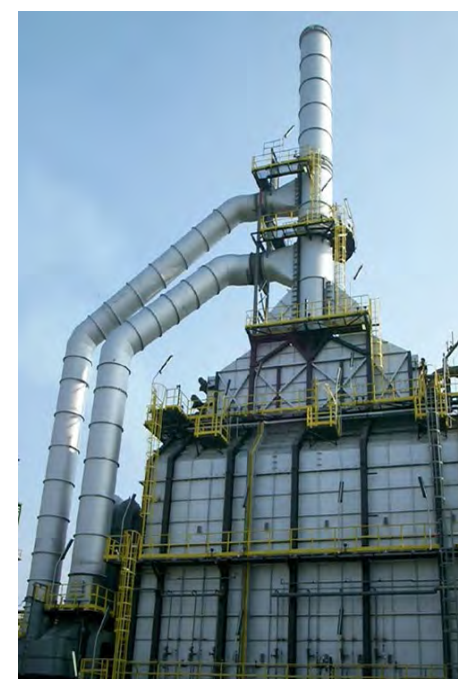
Replacement-of Platforming Furnace
