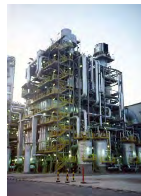
Steam Reformer for 1500 MTPD Ammonia Plant
